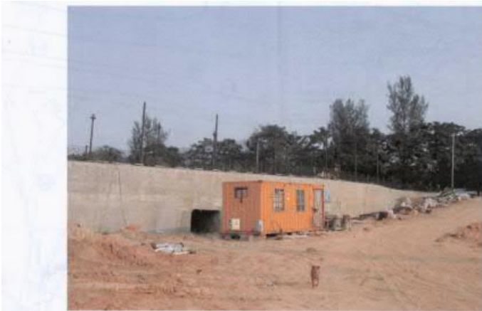
Photo taken on: 22 July 2003 (Front Elevation of the Ramp Structure)
