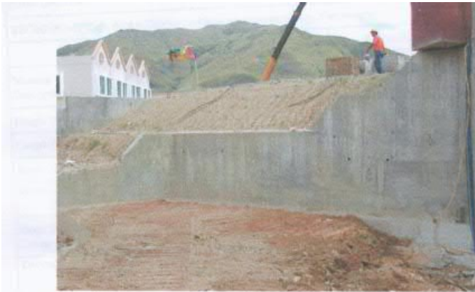
Photo taken on: 22 July 2003 (Front Elevation of RW-2)
