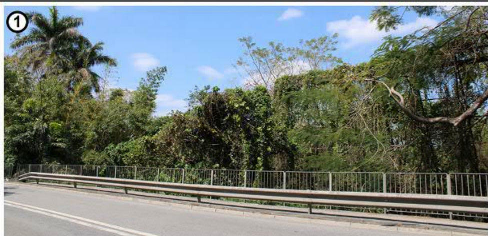
Existing View of Site 1 from Kam Tin Road
